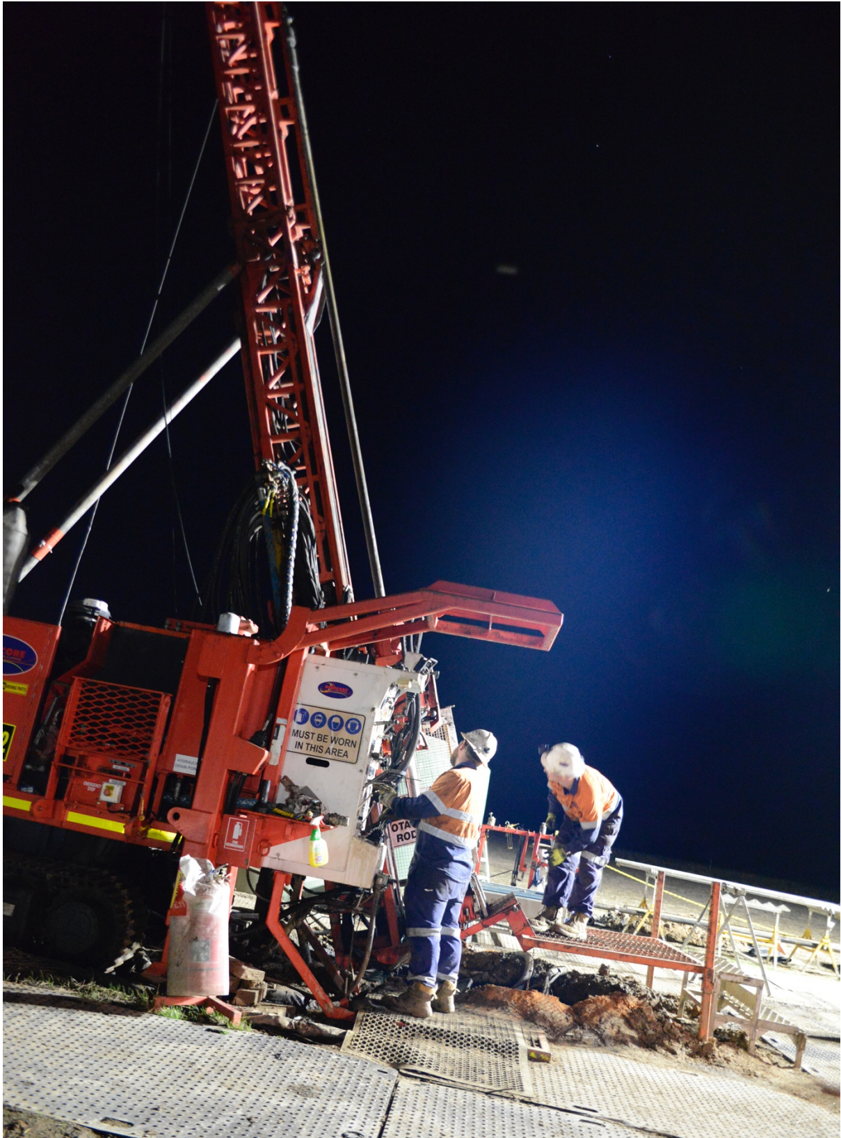
Fig8. Night drilling at Wildwood
