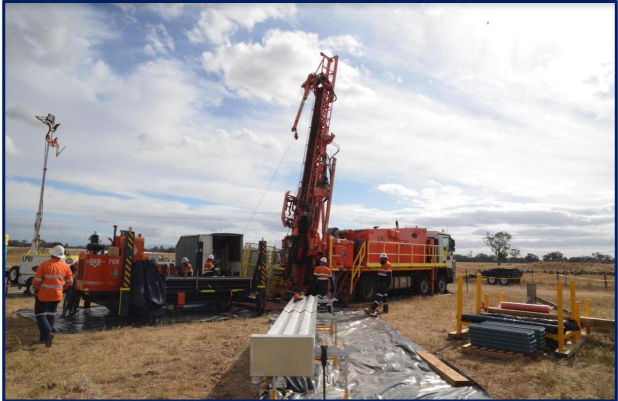
Deepcore Drilling Pty Ltd's Drill Rig onsite at Wildwood Prospect
